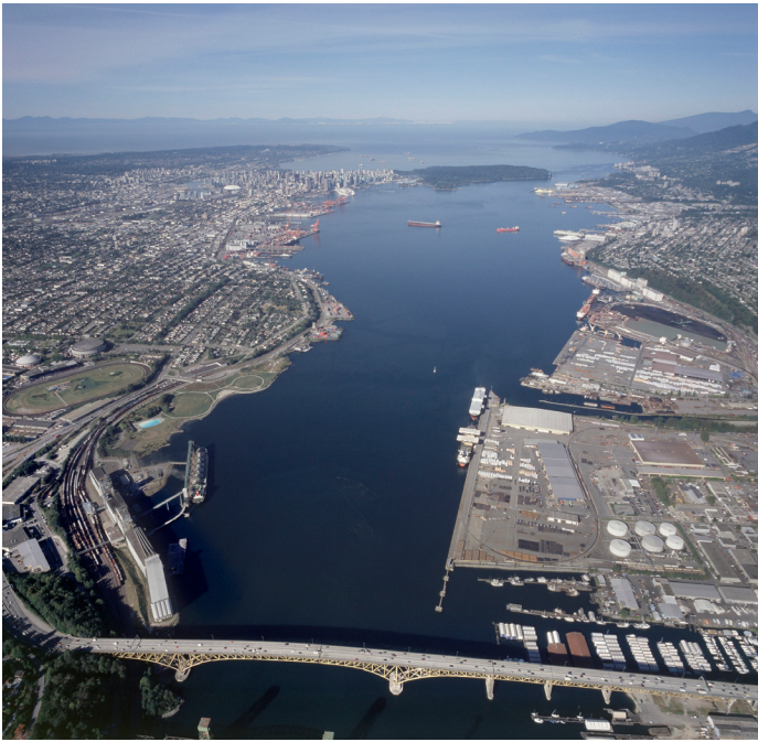
PHOTO: PORT OF VANCOUVER
